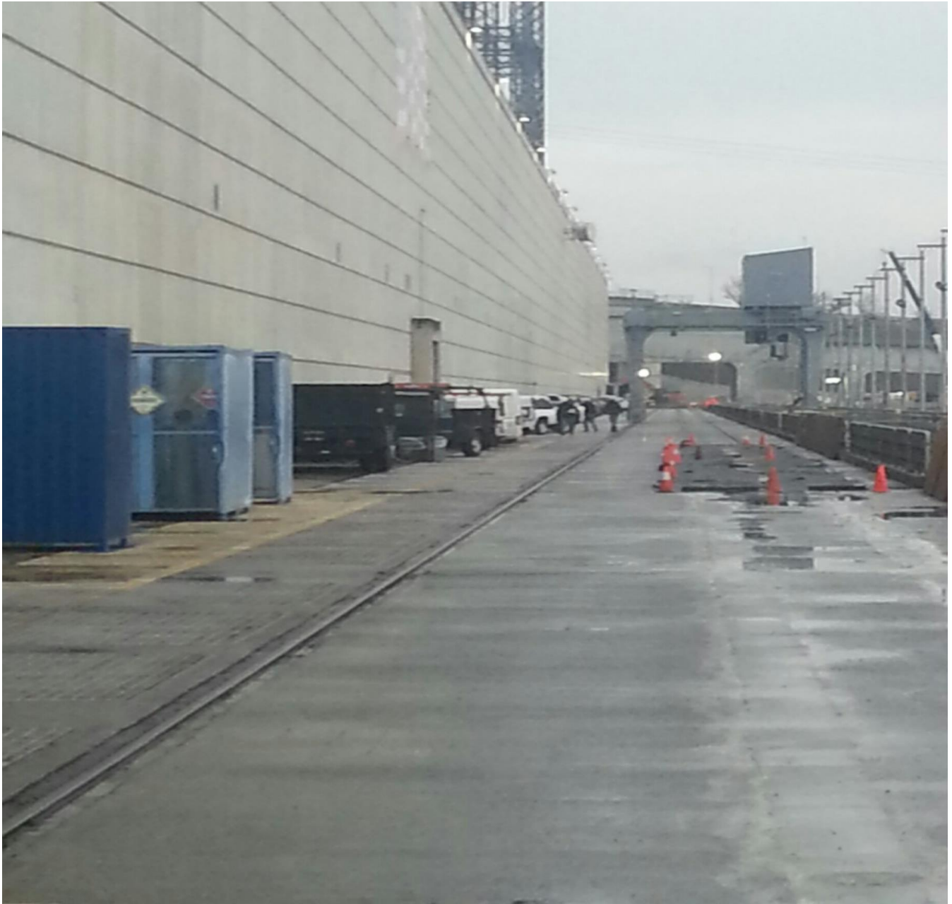
Half done with powerhouse deck rail removal.
